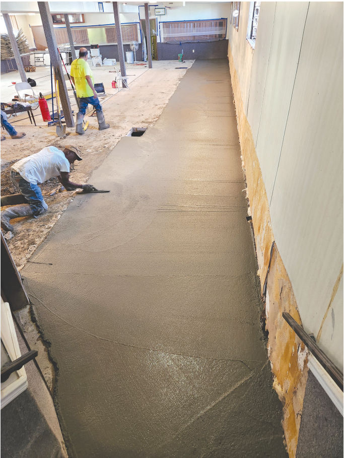
Pictured to the right is the main Blue Room area with the new cement poured where the floor was broke up and heaving with the north wall to yet be sheet rocked.
